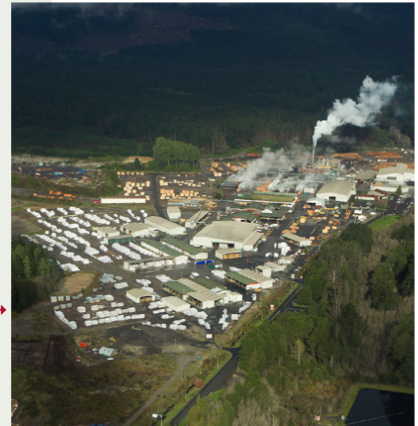
Red Stag Sawmill and processing plants located in Waipa Valley, Rotorua, New Zealand →
